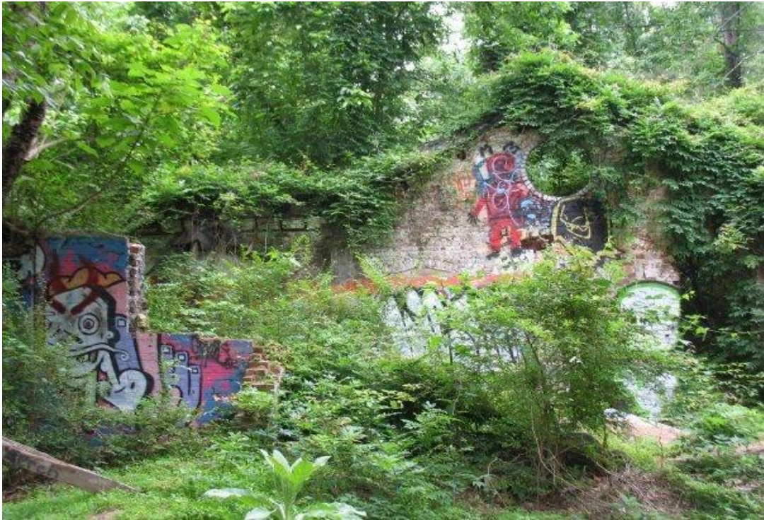
The Decatur Waterworks
